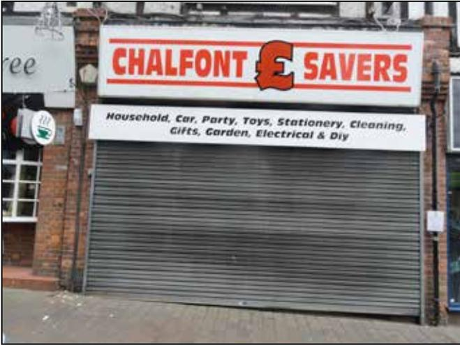
Fig 2.6: Unacceptable solid external shutter
